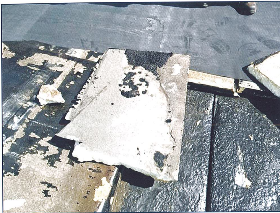
Figure 8 – Substandard adhesion of insulation over tees has been encountered in a number of instances. Concrete is a thermal sink and can become very cold, so direct mopping of hot asphalt should embody long-recognized cold-weather procedures. Note also the lack of taped decking joints.
