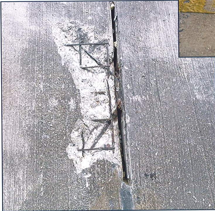
Figure 7 – Whether the cracking or corrosion starts first, the combination makes connection brackets prone to damage. When investigating tees, exploratory openings are crucial to evaluate the condition of brackets.
