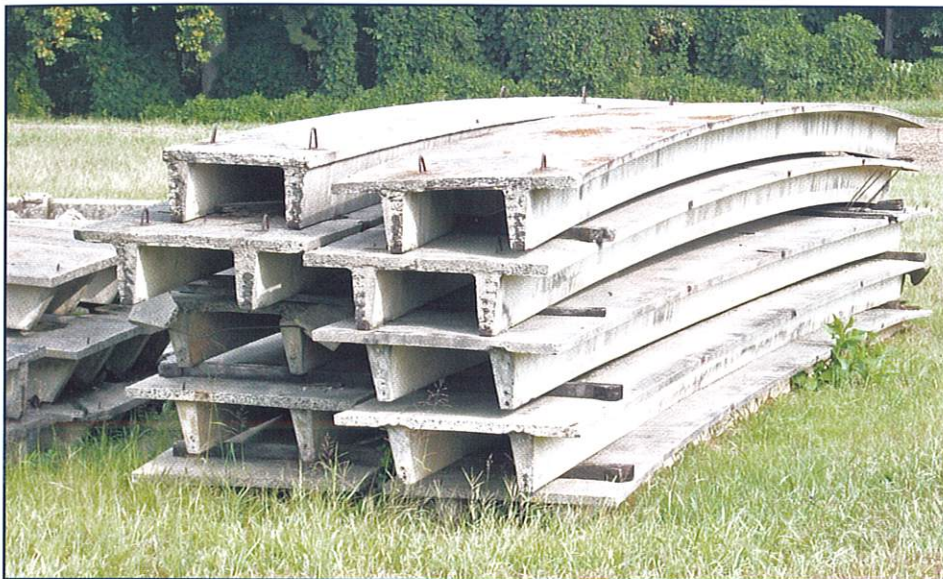
Figure 3 – Camber of tees from compression induced by the embedded prestressing tendons. This is beneficial to counteract the dead-load, live-load, and creep deflection of panels.
