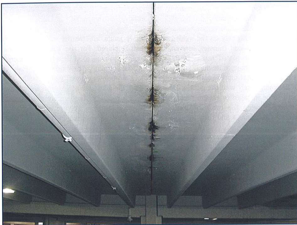
Figure 5 – Parking deck joints are particularly prone to leakage. Backer rods cannot be properly installed at the embedded connection brackets, and the joint geometry makes them susceptible to failure.
