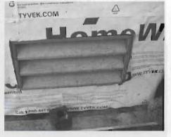
In order for an air barrier to be effective, all of its penetrations and seams would have to be sealed. Lack of flashing around this louver will also render this air barrier ineffective if it is intended to serve as a weather-resistive barrier. Also note that the sheet material has been stapled to the substrate and its seams are not taped. Stapling the membrane to the substrate typically does not provide adequate resistance to wind pressure.
