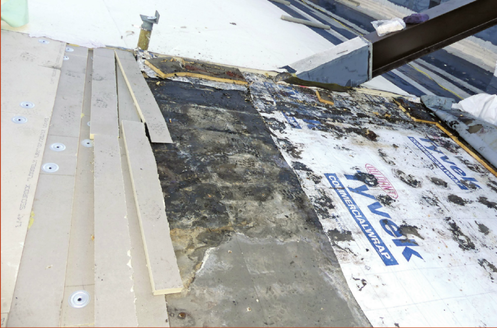
Figure 11. Tear-off in progress at lower dome. Note the signs of moisture on the existing insulation.
