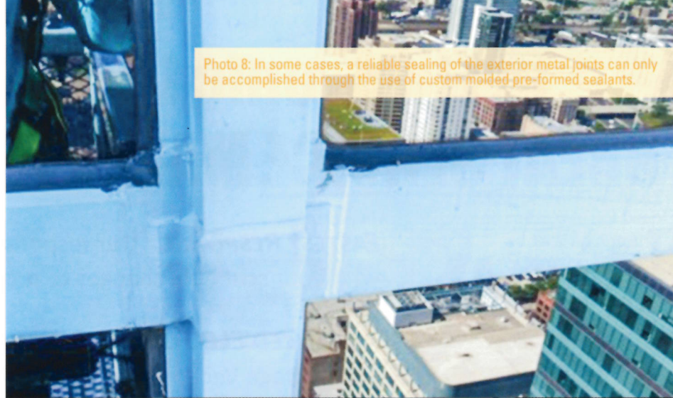
Photo 9: The use of custom molded pre-formed sealants at a curtain wall system. Note that not only the shape, but also the color have to be customized for a project. Such joints can become unsightly once they collect airborne dirt.
