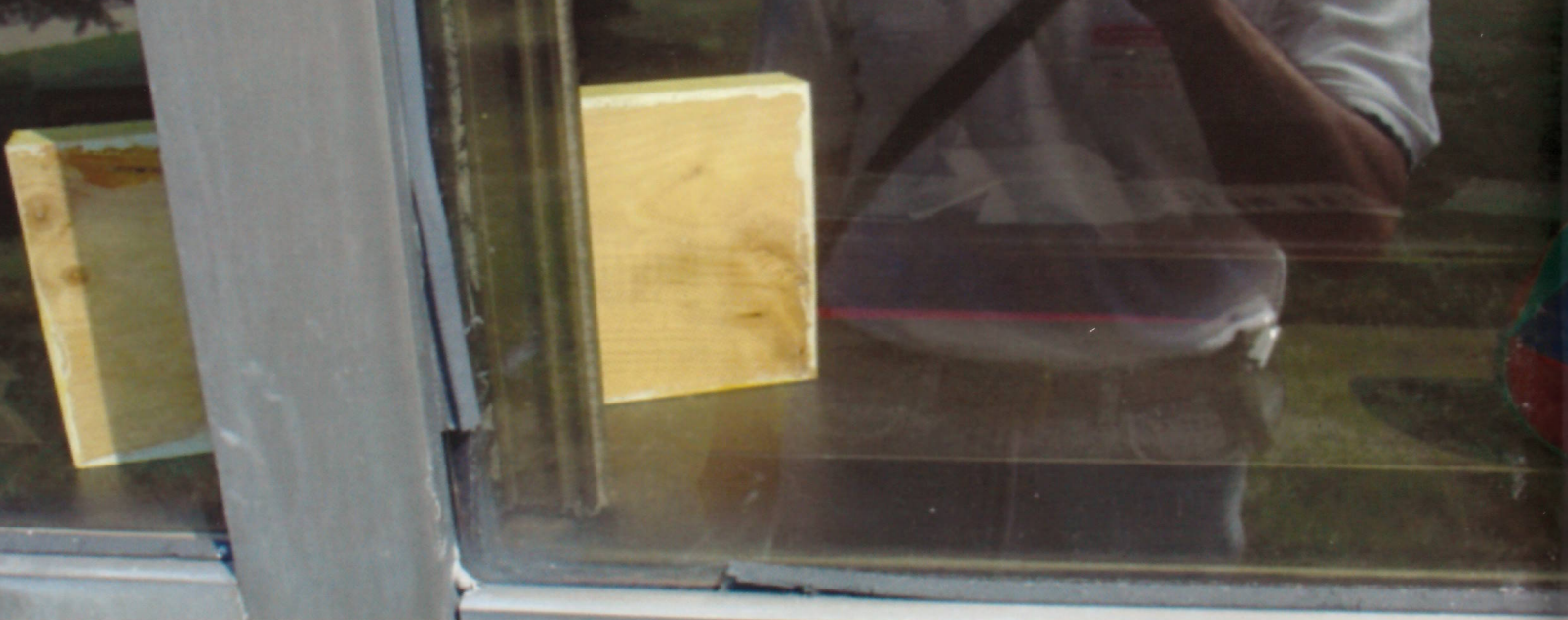
Photo 2: Extensive shrinkage and deterioration of glazing gaskets.
