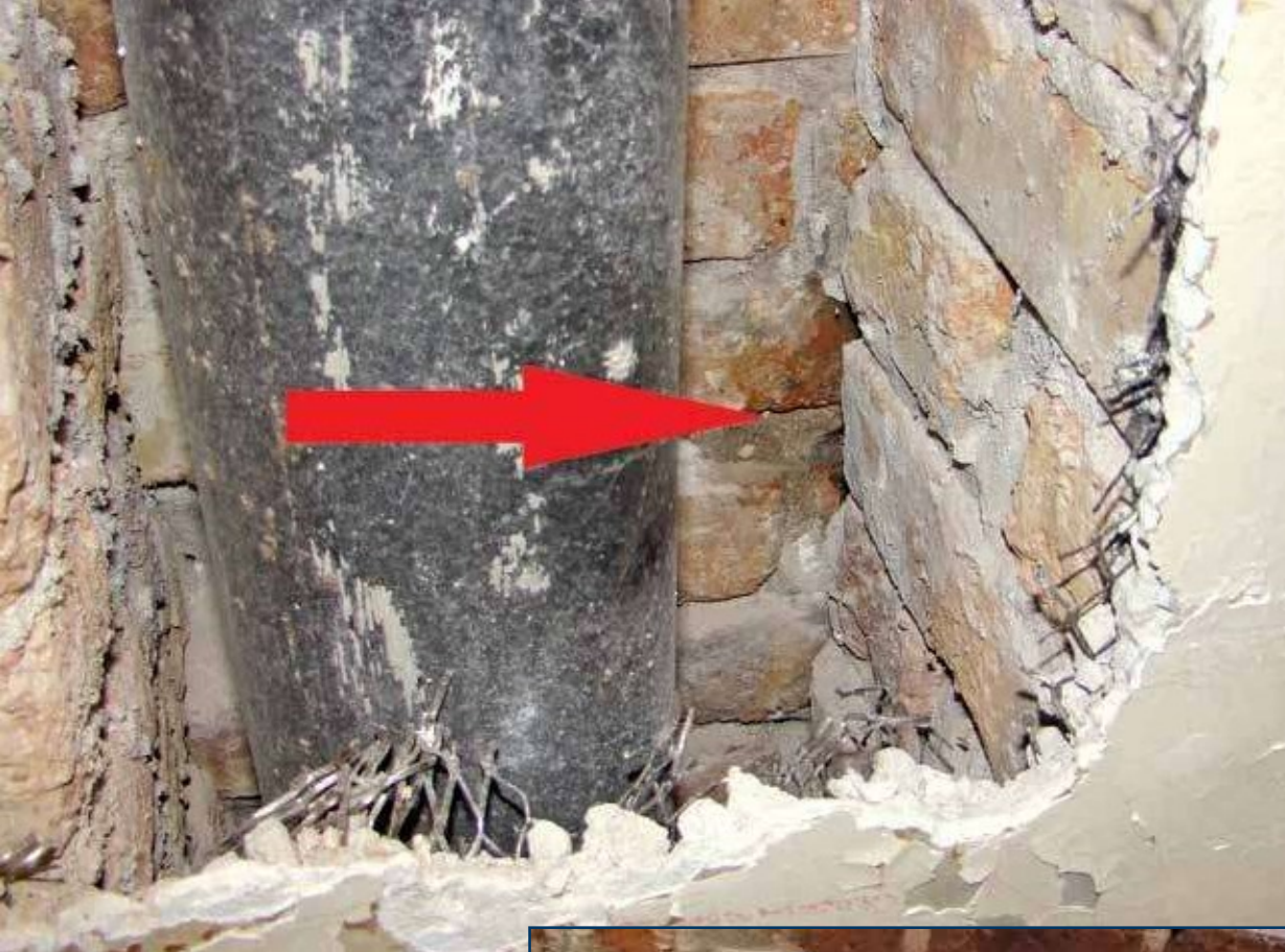
Photo 3 – Leak location at wall section reduced from four- to two-brick masonry wythes to accommodate internal drain pipe.
