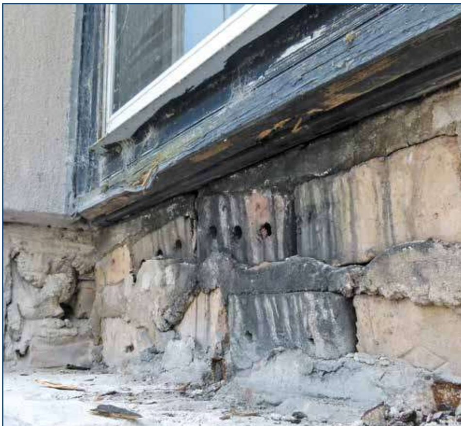
Photo 10 – Staining on backup brick masonry indicates water travel path through wood windowsill into masonry wall.
