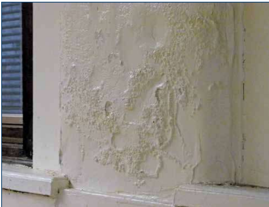
Photo 6 – Deterioration of interior gypsum-based plaster finishes.
