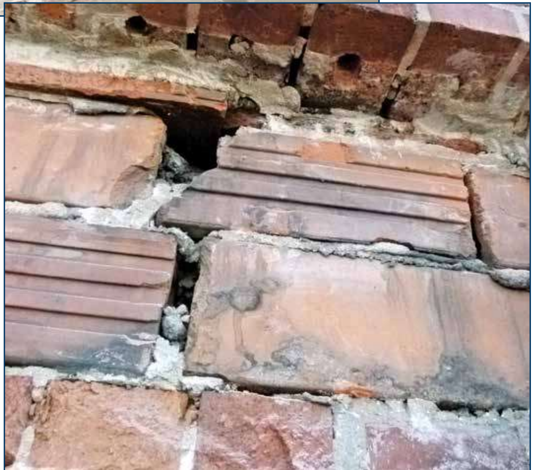
Photo 4 – Use of hollow clay tile units as backup wythes reduces the mass of masonry that can absorb and retain moisture.
