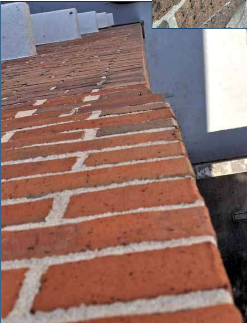
Photo 2 – Parapet wall lateral displacement due to inadequate accommodation of irreversible expansion of the brick masonry.
