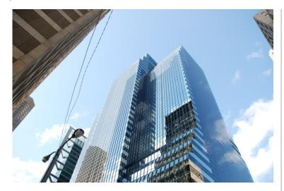
Citigroup Center is a 40-story steel and concrete frame building with a continuous glass and aluminum curtain wall. There are several roof levels on the building. Typical roofing system consists of a split slab assembly with an EPDM waterproofing system. The 40<sup>th</sup> floor includes a large mechanical roof surrounded by a 3-story tall curtain wall system that is exposed on both sides.
