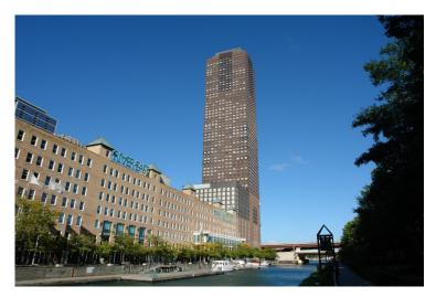
The 474 North Lake Shore Drive building is a 61-story, 505-unit, multi-family condominium building. The building was constructed as apartments in 1990 and converted to condominiums in 2005. The building's exterior is clad with precast concrete panels and aluminum frame windows. The first 15 floors of the building consist primarily of a parking garage. The parking garage facade includes precast concrete louvers in lieu of windows.
