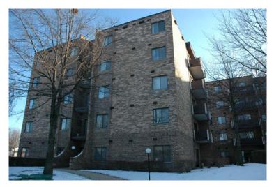
Village on the Lake Condominiums consists of several large 5story buildings which form a residential community. Each building is constructed on perimeter concrete footings and foundation walls. The exterior walls are primarily constructed of load-bearing masonry. The floors consist of concrete on metal deck, supported by steel joints and beams.
