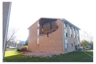
The Glen Manor Condominium Association consists of six 3-story wood-framed buildings constructed in about 1980. The exterior walls primarily consisted of brick masonry that was anchored to wood studs with corrugated galvanized steel ties. Gravity support of the walls was only provided at the building foundation. The exterior walls also included vertical strips of windows and siding panels.
