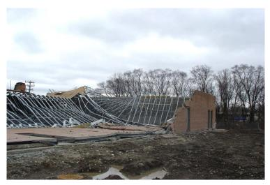
The Wildbrook Development consists of two 12,000-square-foot commercial buildings. Each building consisted of a single-story structure with a steep slope roofing system. The buildings were clad in brick masonry over partially grouted concrete masonry load-bearing back-up walls. The roof assembly consisted of light-gauge galvanized steel trusses, oriented strand board sheathing, and asphalt shingles.
