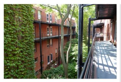
Hedgerow Condominiums is a residential complex consisting of two 4-story buildings. Exterior walls consist of load-bearing masonry walls. Interior floors are generally framed with openweb wood trusses.
