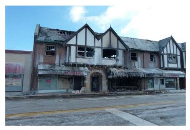
The historic Busse Building in downtown Mount Prospect was a 2-story structure built in the early 1920s. Timber roof and floor framing was supported on masonry bearing walls. The building contained a restaurant, the Chamber of Commerce, a realty company, and 6 upper-level residential units.
