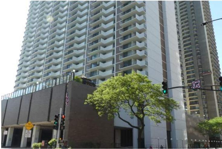
The Malibu East Condominium Building is a 45-story concrete frame structure completed in 1972. The lower 4 floors primarily consist of common building areas, a parking garage, and a few residential units. The east side of the development abuts Lake Michigan. There is a driven steel sheet piling wall with a cast-in-place concrete cap (sea wall) that forms a parapet separating the elevated access drive from Lake Michigan. This area is referred to as the boat dock.
