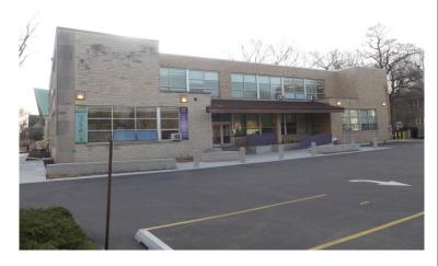
Built in the 1950s, the Beth Emet Synagogue is an approximately 25,000 square foot religious facility. The exterior walls of the 2-story structure are primarily clad with limestone. The roofing systems are comprised of a combination of low-slope and steep-slope roofs. The low-slope roofs are covered with a modified bitumen membrane roofing system over a poured gypsum deck. The eastern portion of the facility consists of steep-slope roofs covered with standing seam copper panels.
