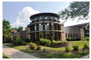
The Woodstock Public Library is a 2-story structure clad with brick and stone masonry, and with horizontal cedar siding. The roofs consist of steep-slope and low-slope roofing systems. The steep-slope roofs are covered with 3-tab asphalt shingles. The low-slope roofs are covered with a mechanically attached thermoplastic roof membrane over rigid insulation and structural steel roof deck.
