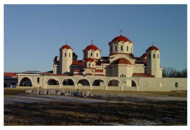
The new St. John Monastery campus consists of several buildings including the church building that was designed to replicate the old Greek orthodox churches of the 16th century. The new church building included several domes, gable and hip roofs, and arch barrel roofs. The dome roofs include geometrically complex shapes that required extensive computer modeling.
