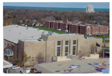
McGaw Memorial Hall is a steel frame structure that serves as Northwestern University's basketball arena. The building has 8 separate roof sections. The largest roof section consists of a gable roof that covers the majority of the arena and measures approximately 60,000 square feet in plan.
