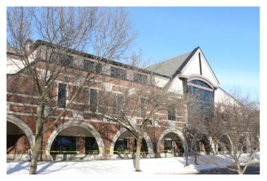
Glen Ellyn Public Library is a 3-story steel and wood frame building originally constructed in 1995. The building roofs are steep-slope with asphalt shingles. Exterior walls at the library are primarily clad with brick masonry veneer, cast stone, and exterior insulation and finish system (EIFS). Large aluminum and glass curtain walls are located at the east, south, and west elevations. Existing windows are aluminum frame with insulated glazing panels.
