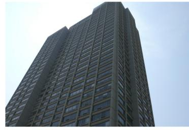
1700 East 56th Street is a 40-story concrete frame building built in the 1960s. There are several roof levels on the building. The main roof level over the top-floor units consists of 3 separate sections. The middle section was originally designed as a sundeck with a concrete topping slab. The east and west sections of the roof have a conventional roofing system. In addition to the main level roofs, there are approximately 4 additional penthouse roofs, all located above the main roof level.
