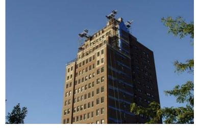
Located at 5510 North Sheridan Road, The Renaissance Building is a 17-story high-rise completed in 1928. The building is concrete framed and clad in brick and limestone masonry.
