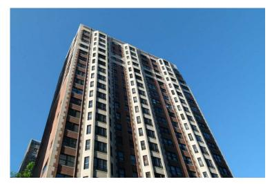
Eddystone is a 22-story building originally constructed in 1927. The building structure consists of reinforced concrete floorslabs supported by structural steel and concrete framing. The exterior walls are clad in brick and limestone masonry.
