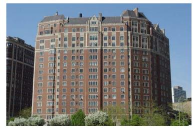
The 3800 North Lake Shore Drive Building is a 17-story high rise completed in 1927. The building is concrete framed and clad in architectural terra cotta, brick, and limestone. The limestone units on the building are not original. They were used to replace terra cotta during previous repair projects. The mansard roofs include terra cotta clad chimneys and dormers with large finials.
