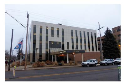
Built in 1985, the Riverside Park Plaza building is a 5-story medical office building. It is a steel-framed structure, with its facade originally clad with a portland cement plaster (stucco) system over gypsum sheathing and cold-formed steel stud walls.
