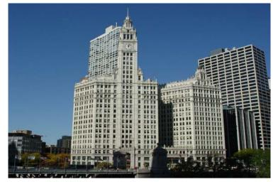
The Wrigley Building consists of two towers, a breezeway connecting the two towers at grade, and a sky bridge between the two towers at the 14<sup>th</sup> floor. The South tower rises 28 stories above Upper Michigan Avenue and was completed in 1921. The North Tower was completed in 1924.
