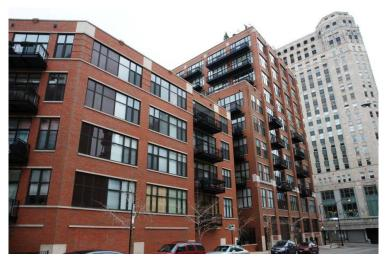
The Union Square Condominium Association consists of a 5-story building completed in 1998 and a 10-story building converted from an existing factory at the same time. During the conversion, an additional 4 stories were added to the existing 6-story factory that was originally constructed in 1918 and expanded in 1938 and 1946.
