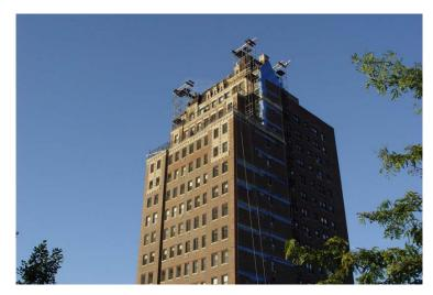
Located at 5510 North Sheridan Road, The Renaissance Building is a 17-story high-rise completed in 1928. The building is concrete framed and clad in brick and limestone masonry.
