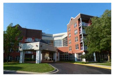
The Moorings of Arlington Heights is a retirement community that includes a 5-story concrete-framed building, clad in brick masonry. The 5-story lobby atrium is enclosed by vertical and sloped glazing systems. Water leakage through the vertical glazing system had been an ongoing problem for many years, despite several attempts to address the leaks.
