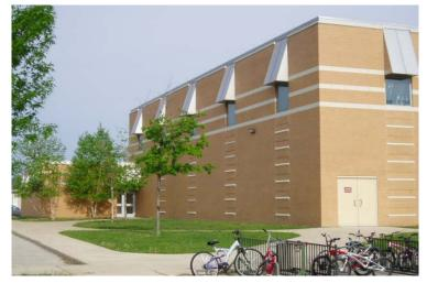
Shabonna Middle School is a 2-story steel frame building with masonry cavity exterior walls. These walls consist of a brick veneer, a drainage cavity, extruded polystyrene insulation, and CMU back-up.
