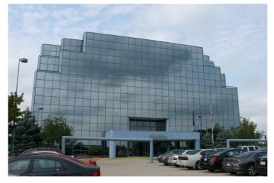
Naperville Financial Center is a 5-story steel frame commercial building constructed in 1986. The building features a glass and aluminum curtain wall facade, with several set-back patios at the upper 2 levels of the building.
