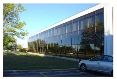
The Motorola Parts Building in Motorola's Schaumburg, Illinois, campus is a large office/manufacturing facility built in the 1960s. The office wing of the building is a 2-story steel frame building with an aluminum/glass curtain wall system on 3 sides. The curtain wall system consists of insulated vision glass and spandrel panels.
