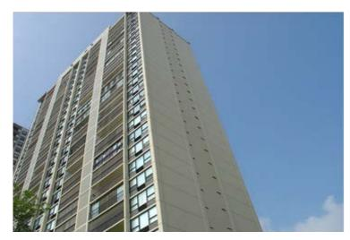
Horizon House Condominiums is a 30-story concrete frame building that was constructed in 1963. The windows at the building consist of redwood frame windows with single pane glass panels, and aluminum frame operable hopper windows that were installed in the wood frames.
