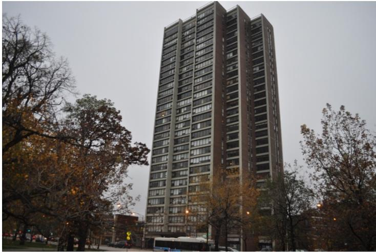
The Hemmingway House Condominium Building is a 30-story concrete frame structure completed in 1969. The exterior facade of the building consists of exposed concrete columns, slab edges and beams; infill brick masonry walls, and aluminum frame windows. The Association requested that BTC evaluate the condition of the exterior walls and windows; and identify potential causes of systemic interior water leakage.
