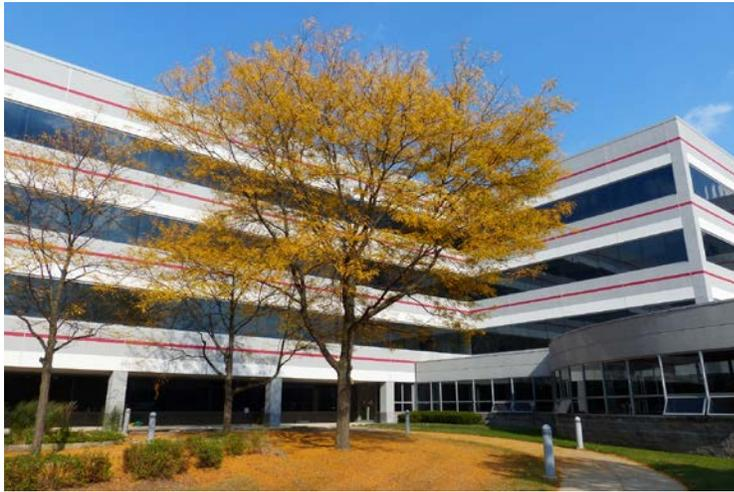
Fisher Corporate Center is a 4-story office building constructed in 1992. The building was primarily clad in 6,400 linear feet of prefabricated exterior insulation and finish system (EIFS) panels and aluminum frame strip windows. Water leakage throughout the facade began shortly after construction.
