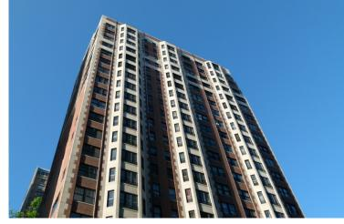
Eddystone is a 22-story building originally constructed in 1927. The building structure consists of reinforced concrete floor slabs supported by structural steel and concrete framing. The exterior walls are clad in brick and limestone masonry. Persistent water leaks were an ongoing problem at the building for many years. Eddystone retained BTC to evaluate the building facade and provide recommended options for repairs.
