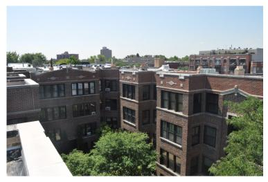
The 743 through 755 West Brompton Condominium Association consists of a 3-story courtyard building constructed circa 1920. The exterior walls are generally constructed of triple-wythe load-bearing brick masonry, and include limestone accents and crenellations near the top of the walls.
