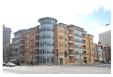
The building is a 6-story structure built in 2006. The turret at the northeast corner and portions of the north and east elevations are clad with a composite metal panel (CMP) cladding system and aluminum framed windows.
