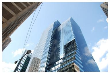
Citigroup Center is a 40-story steel and concrete frame building with a continuous glass and aluminum curtain wall. There are several roof levels on the building. Typical roofing system consists of a split slab assembly with an ethylene propylene diene monomer waterproofing system. The 40<sup>th</sup> floor includes a large mechanical roof surrounded by a 3-story tall curtain wall system that is exposed on both sides.
