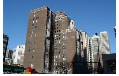
The 20 East Cedar Building is a 19-story gothic high rise completed in 1925. The center of the building steps back at the south elevation to form terraces at the 14<sup>th</sup> and 18<sup>th</sup> floors. The building is concrete framed and clad in brick and architectural terra cotta. The south elevation also includes four 2-story terra cotta clad Oriel windows, a projecting terra cotta clad spiral stairway enclosure, and 7 large finials at the 14<sup>th</sup> floor terrace.
