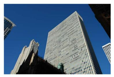
The 111 East Chestnut building is a 57-story concrete-framed structure completed in 1972. Floors 10 through 57 (Tower) include residential condominiums. The lower 9 floors include a parking garage, restaurant, and commercial space.
