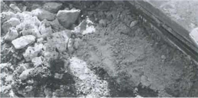
Extensive deterioration of a plaza deck mortar setting bed in a closed joint system. The plaza is located in a cold region.
