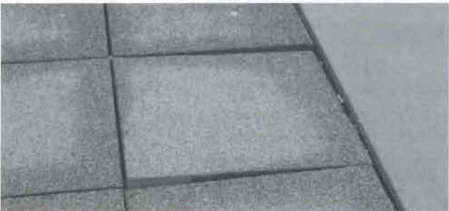
Shifting and rocking of pedestal supported pavers
