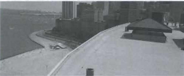
A conventional roof membrane is typically exposed to the environment. Granules or coatings are usually used to UV exposure.
