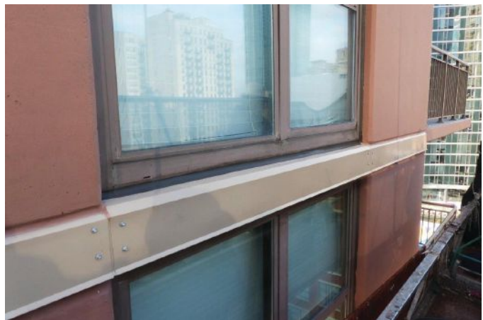
Fig. 7: Slab edge cover at east elevation
