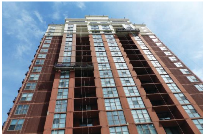
Fig. 8: Swing-stage work on south elevation
