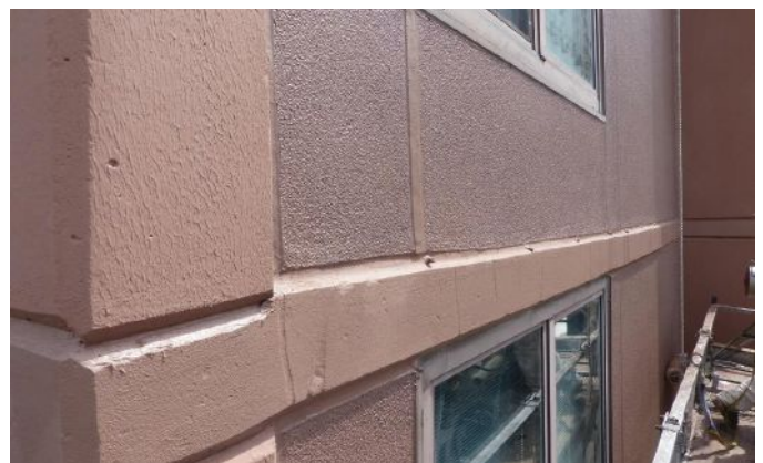
Fig. 5: DEFS crack repair and elastomeric coating; Concrete coating
