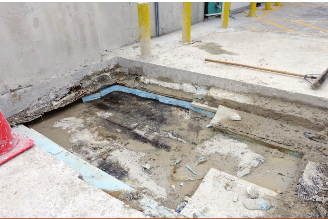
Figure 1. Example of split-slab construction.
