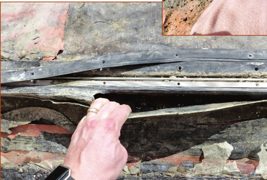
Figure 7. A large tear in an expansion joint flashing sheet.
