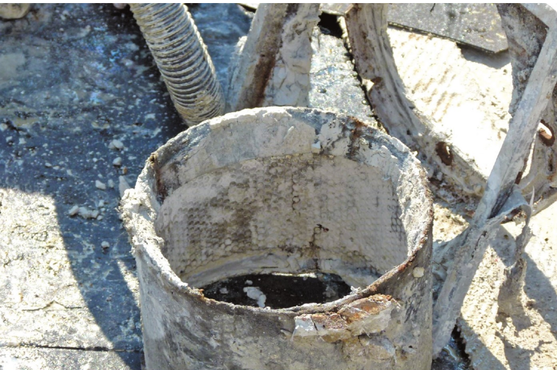
Figure 2. A filter screen around a two-stage drain is clogged due to decalcification of the concrete topping.
