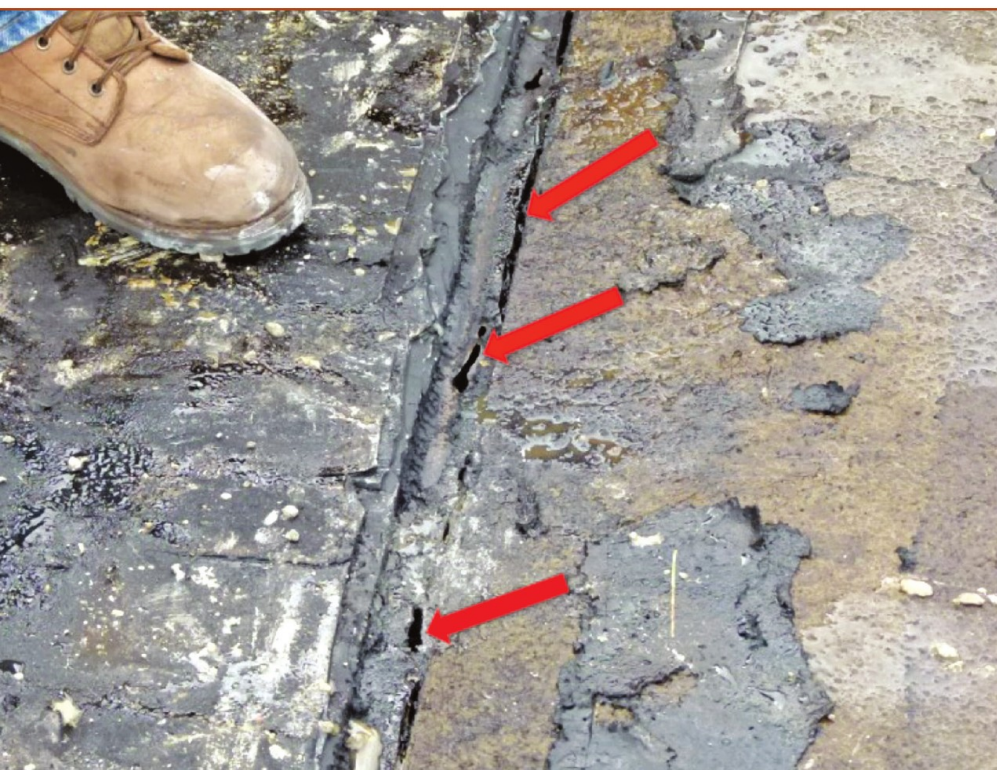
Figure 8. A failed sealant joint.
