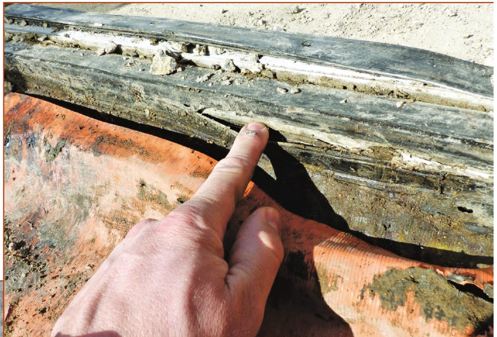
Figure 6. Severed flange of an expansion joint sealing gland.
