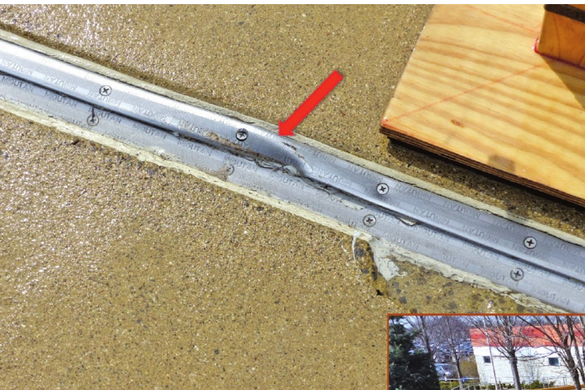
Figure 4. Deformation around a retaining cap.
