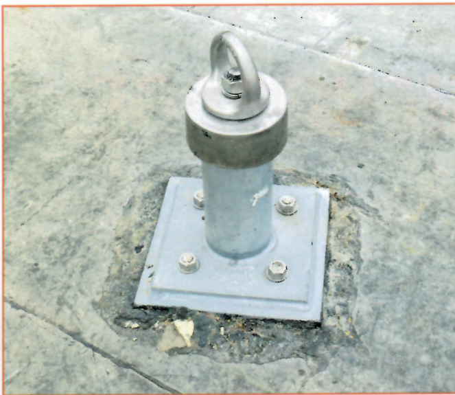
Figure 1 – Proprietary stanchion with a top eyebolt attached to concrete roof deck with adhesive anchors.
