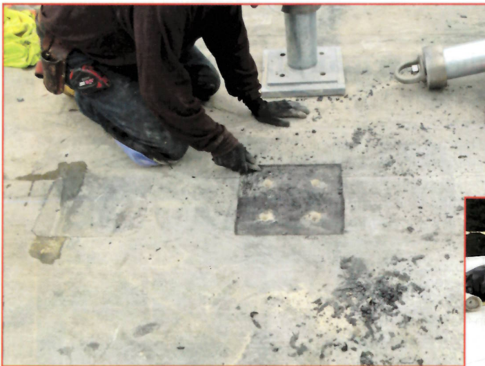
Figure 3 – Vapor retarder removal for fall arrest anchorage directly to concrete roof deck.
