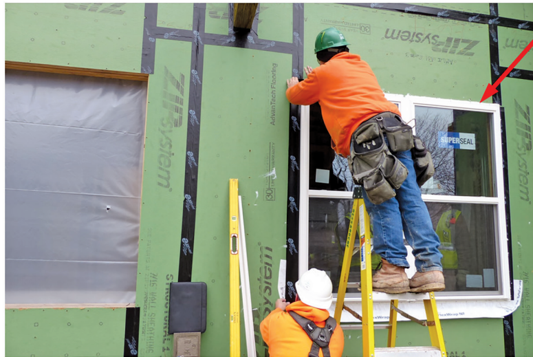
Figure 2 – The second subcontractor involved in the performance of the window installation is the window installer. In this case, the same subcontractor is also responsible for installation of window perimeter flashing.
