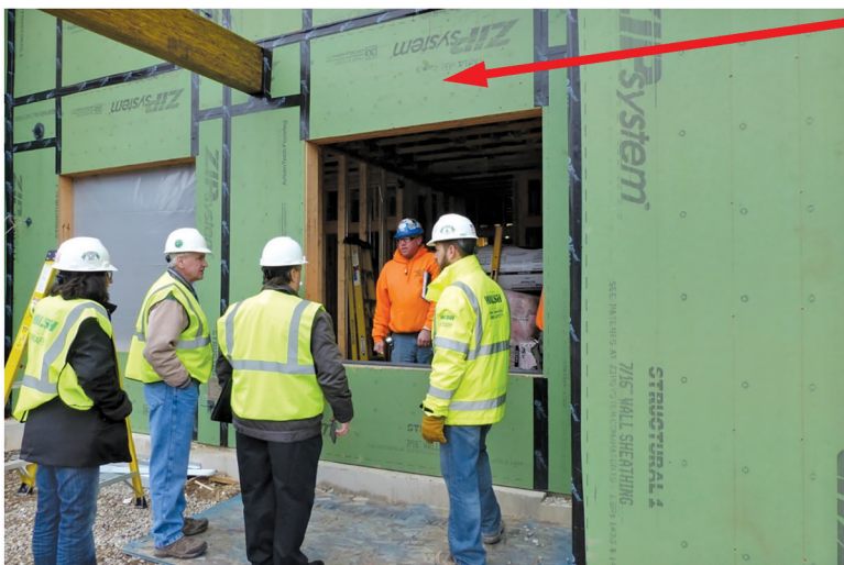
Figure 1 – The first subcontractor indirectly involved in the performance of this mock-up window is the subcontractor who installed the exterior sheathing and air barrier system.
