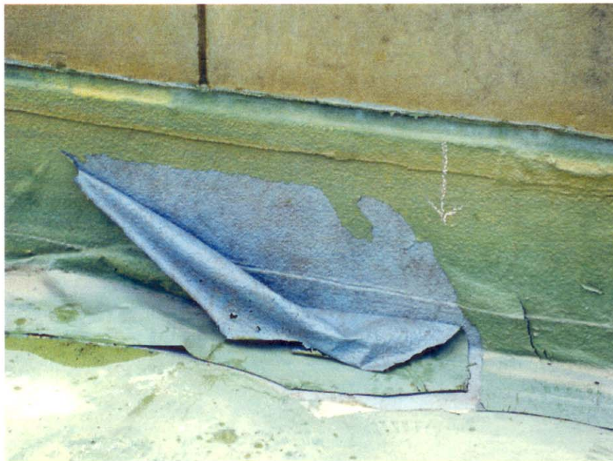
Figure 6 – Large interlayer delaminations of the membrane.
