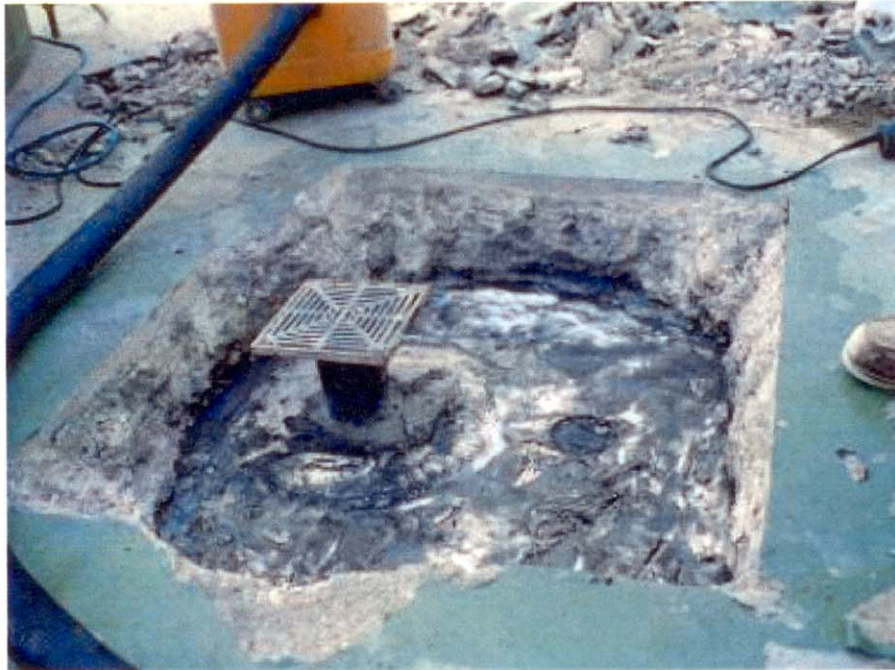
Figure 11 – Overall view of Opening 1 showing the original lead pan and a retrofit drain.
