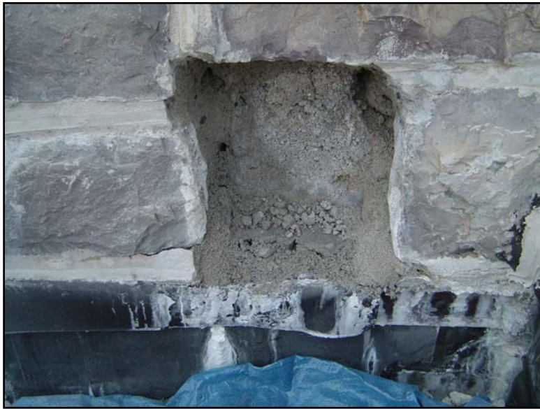
Figure 1. Dry-pack Mortar in Stone Masonry Cavity
