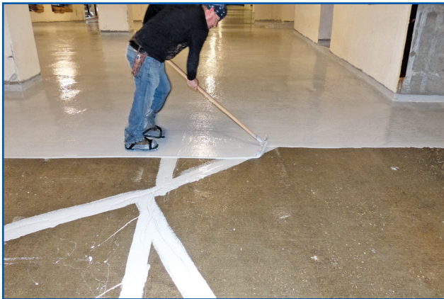
Figure 19 – Base coat application.
