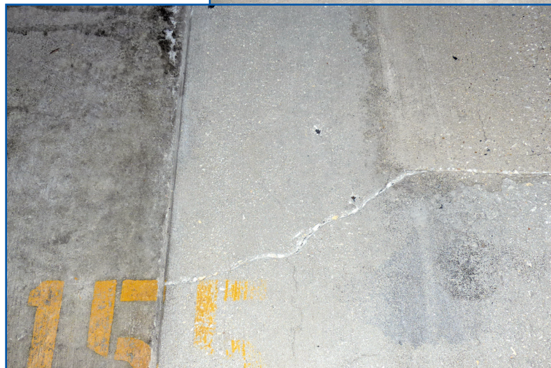
Figure 12 – Shotblasted surface.
