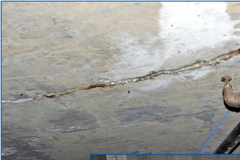
Figure 3 – Moisture migration through slab.
