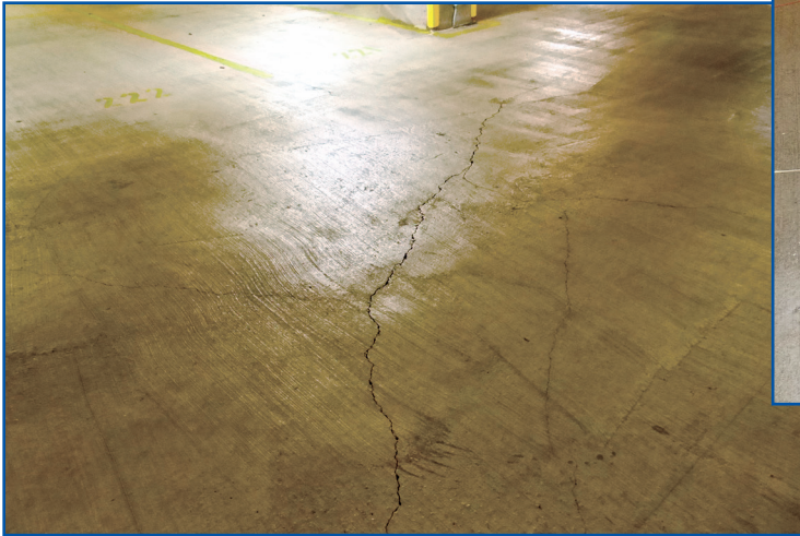
Figure 13 – Cracks in concrete.
