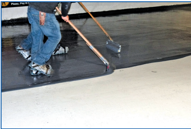
Figure 20 – Intermediate coat application.
