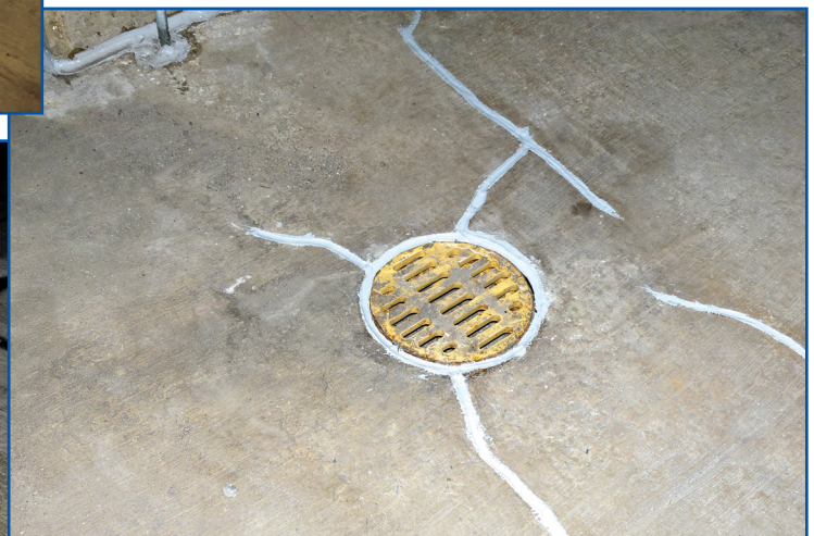
Figure 16 – Sealant at drain perimeter.
