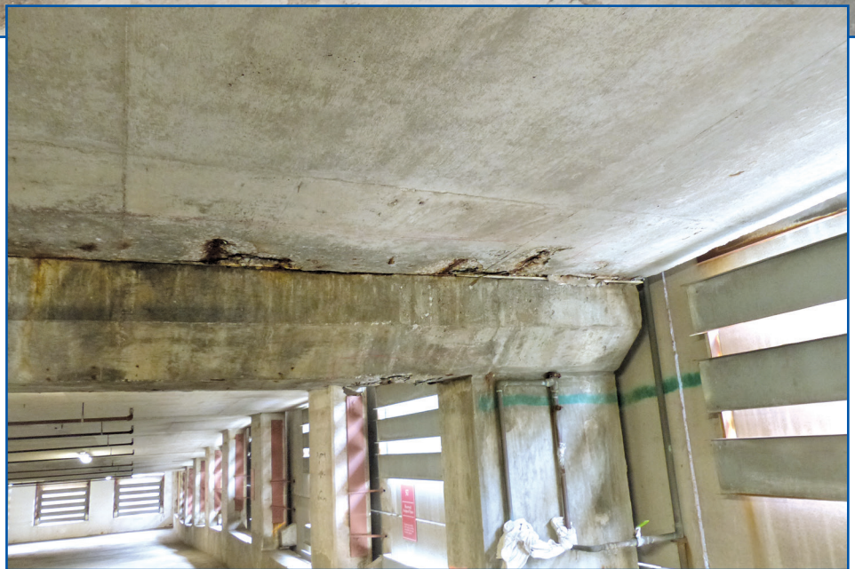
Figure 2 – Corrosion of reinforcing steel.
