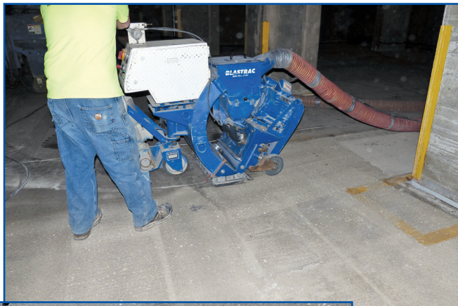
Figure 11 – Shotblasting.
