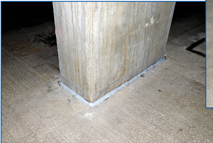
Figure 15 – Sealant at horizontal-to-vertical transitions.
