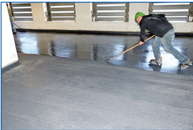
Figure 22 – Finish coat application.
