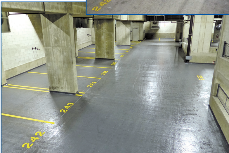
Figure 6 – Parking garage slab after TBM application.
