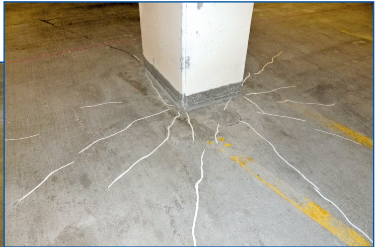
Figure 14 – Routed and sealed cracks.
