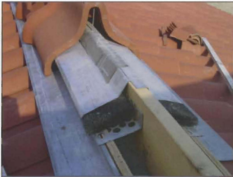
Figure 16 - Roof ridge configuration with ventilation provisions and a lightning arrest rod.
