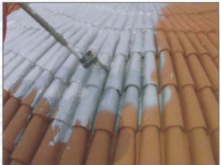
Figure 15 - Application of the elastomeric base coat in all the crevices with a brush.
