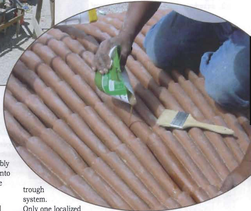
Below: Figure 10 - Sealing of the pie-shaped segment joints with pigmented resin.
