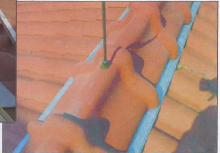
Below: Figure 17 - Roof ridge detail after installation of ridge cap tiles.
