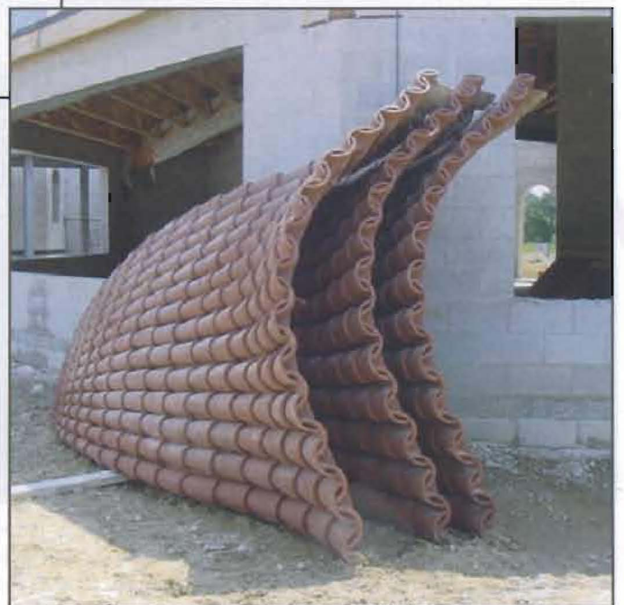
Figure 8 - Outer domes were fabricated and delivered to the site in pie-shaped segments.
