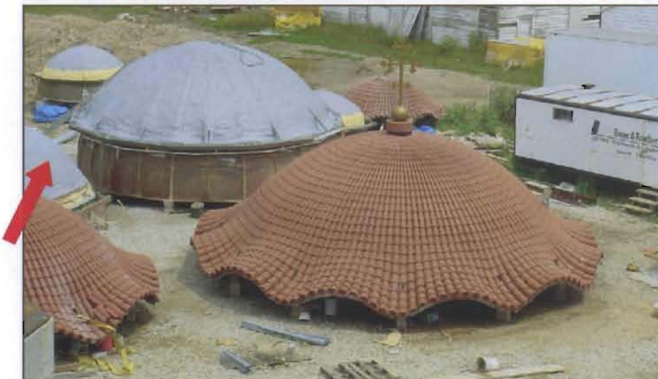
Above: Figure 11 - Assembled inner and outer dome. Note the gray spray polyurethane foam system and the perimeter drain pipes (red arrow).
