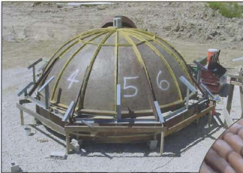
Above: Figure 9 - An inner dome being assembled on the structural steel skeleton.
