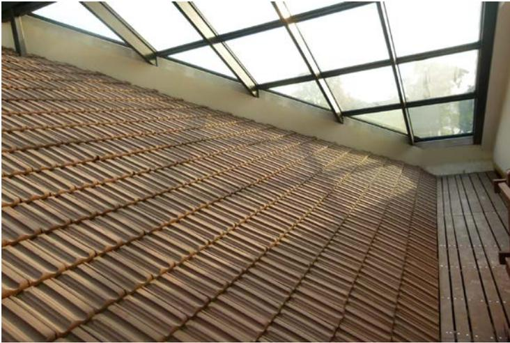
An addition to the Vespasian Warner Public Library building was constructed in 1991. A majority of the roofing system above the original building and addition consists of a steep-slope roofing system covered with clay-tile shingles. As part of the addition, a new skylight system was constructed at the interface between the addition and original 2-story building.
