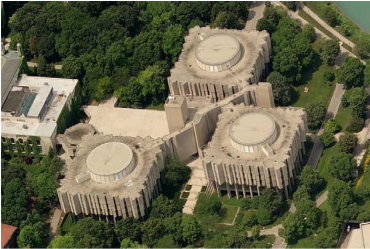
The University Library is a concrete frame structure that serves as Northwestern University's main library. The library consists of 17 low-slope roof sections totaling approximately 60,000 square feet in plan with the largest roof sections being part of the 3 distinctive main towers.
